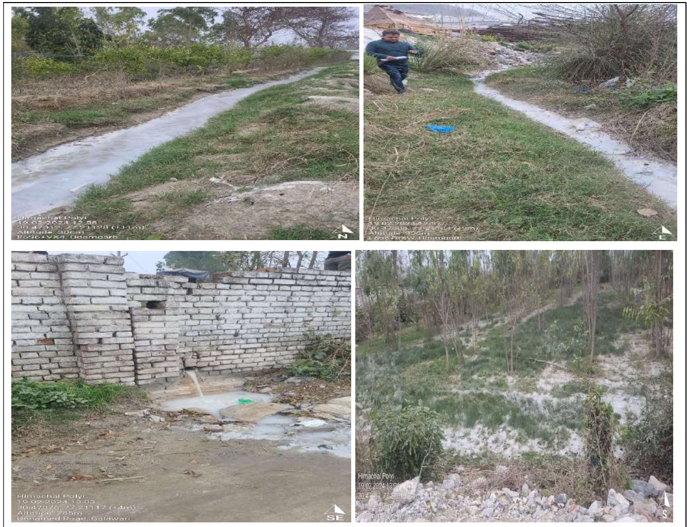
Photographs 18-21: Discharge of effluent in violation of the conditions of CTO
