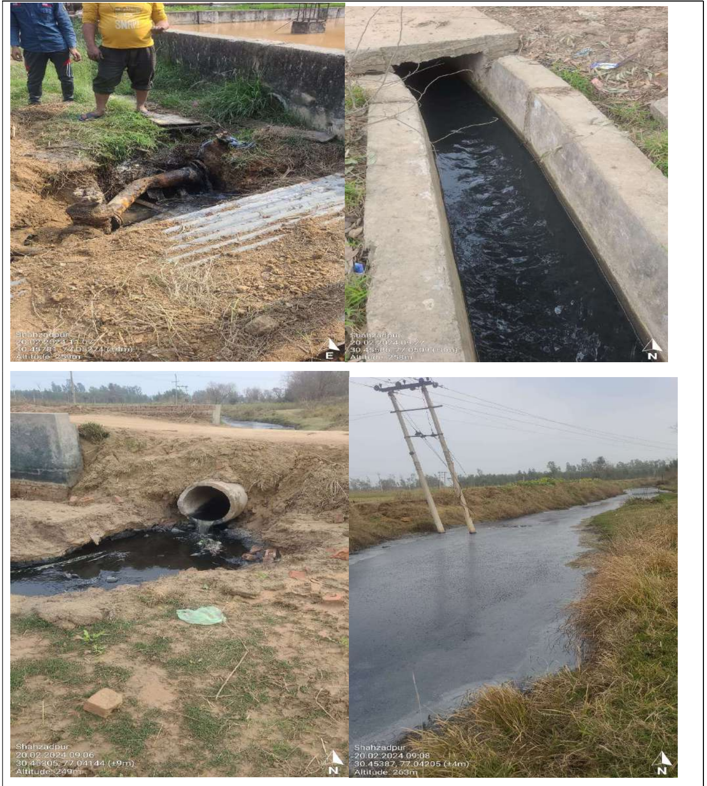
Photographs 22-25: Showing Bypass arrangement made by M/s Naraingarh Sugar Mills Ltd to discharge untreated effluent into the drain leading to river network:
